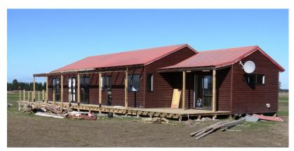
Phase 3 is well under way, comprising the house being tied down to the piles, plumbing connected, ramp and deck almost completed and bathroom/toilet redevelopment progressing well.
