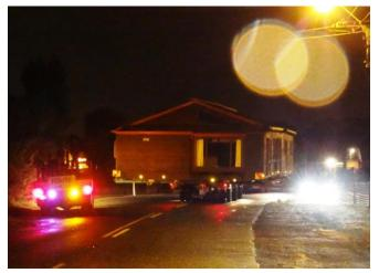
The technology involved was fascinating. The house was lifted on jacks and the "kneeling" trailer eased in under it, raised to take the weight, and progress paused until traffic flow minimised in the wee small hours. Then, under cover of darkness it was driven to our airfield,
