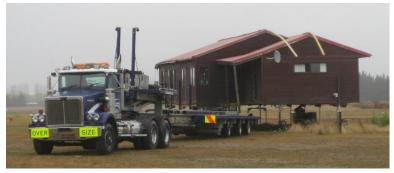
The side jacks were put in place, extended to take the weight, and the trailer knelt down and was eased out from under,
